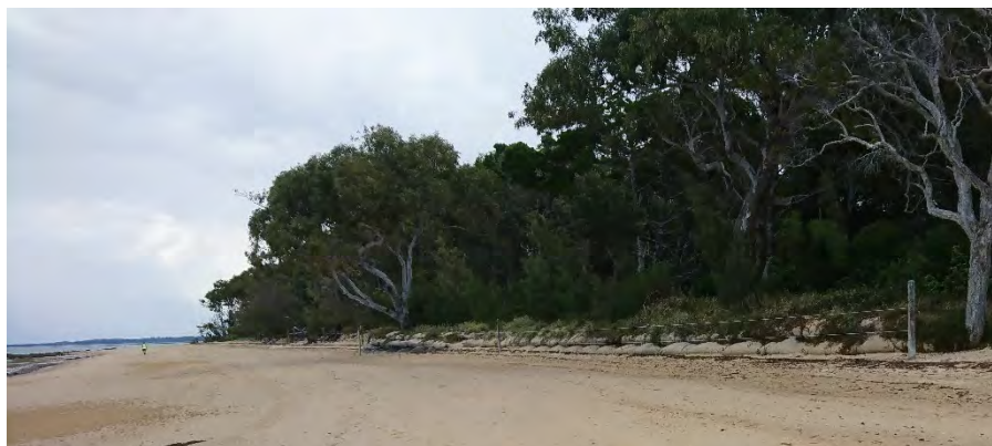
Figure 6-8 Northern geotextile container seawall - October 2018
