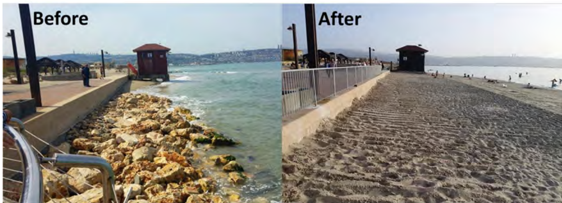
Figure C-3 Beach nourishment before (left) and after (right)
