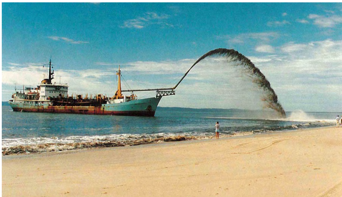
Figure 3-5 Nourishment Sand being Delivered ‘over-the-bow’ to Woorim Beach
