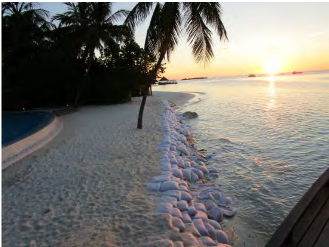
Figure C-6 Eroded beach in front of a geotextile container seawall
