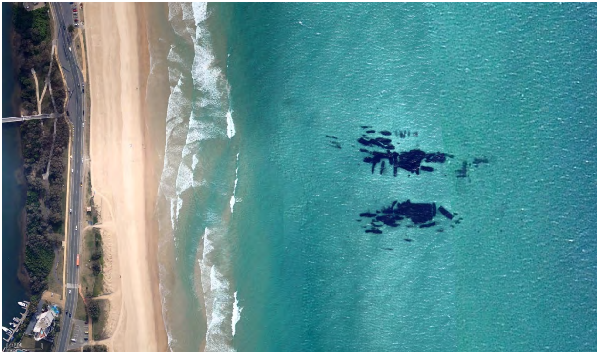
Figure 3-4 Geotextile Sand Container Artificial Reef at Narrowneck, Gold Coast (Source: NearMap, 2011)
